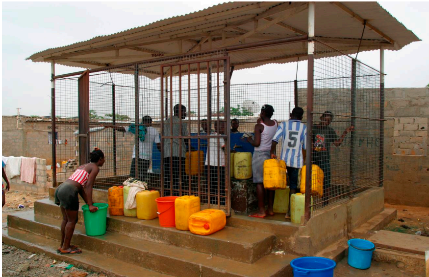
Figure 10. Water kiosks, having six to eight taps, have replaced the stand-pipe mode.
