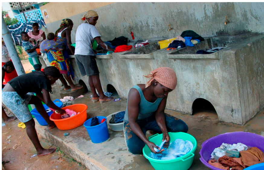
Figure 11. Clothes wash-stands are often installed at the kiosks.
