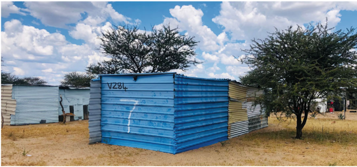
Frame c: Picture showing a closer view of the typical state of housing in the Ekunde 2 Informal Settlement. Despite its poorly serviced substandard housing made of corrugated iron sheets, residents paint their houses colourfully to enhance architectural aesthetics — ©Photograph by authors.
