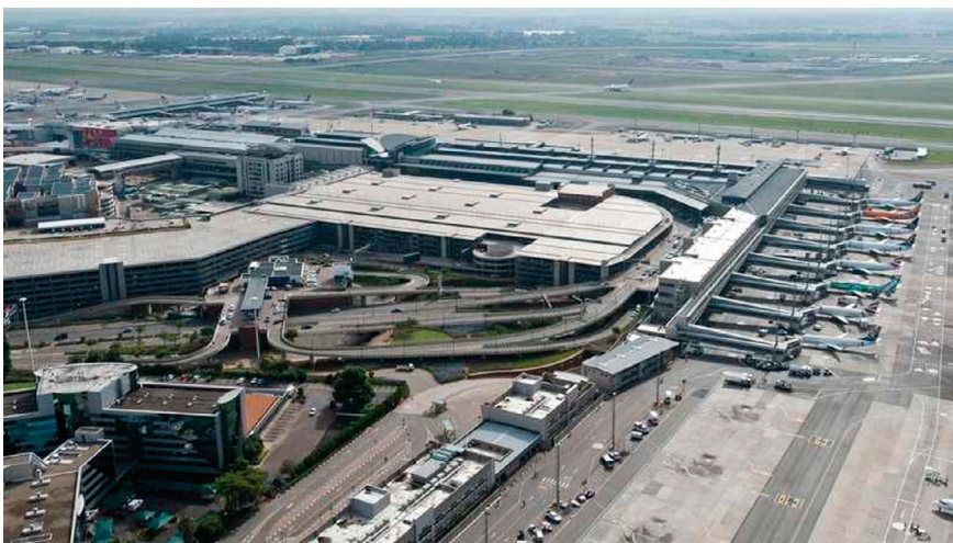
Fig. 9 Aerial view of O.R. Tambo International Airport. Source Tshuma [39]
